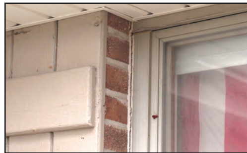
Sealant deterioration
