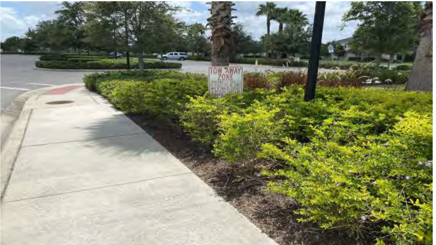
The shrubs need to be trimmed away from the Tow Away sign at the clubhouse parking lot entrance.
