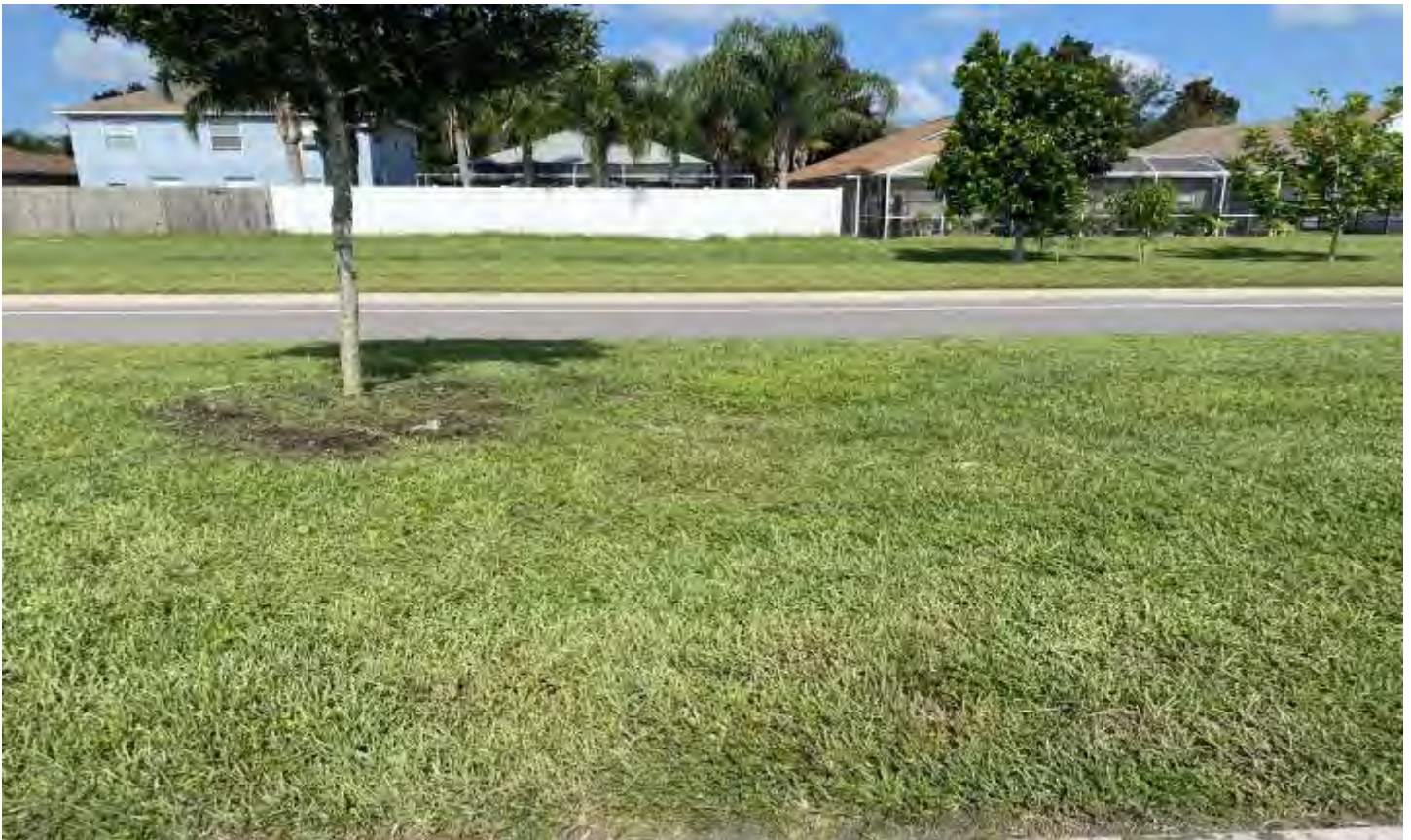
The St. Augustine turf along Summerfield drive is weed infested and tree wells need to be edged and sprayed.
