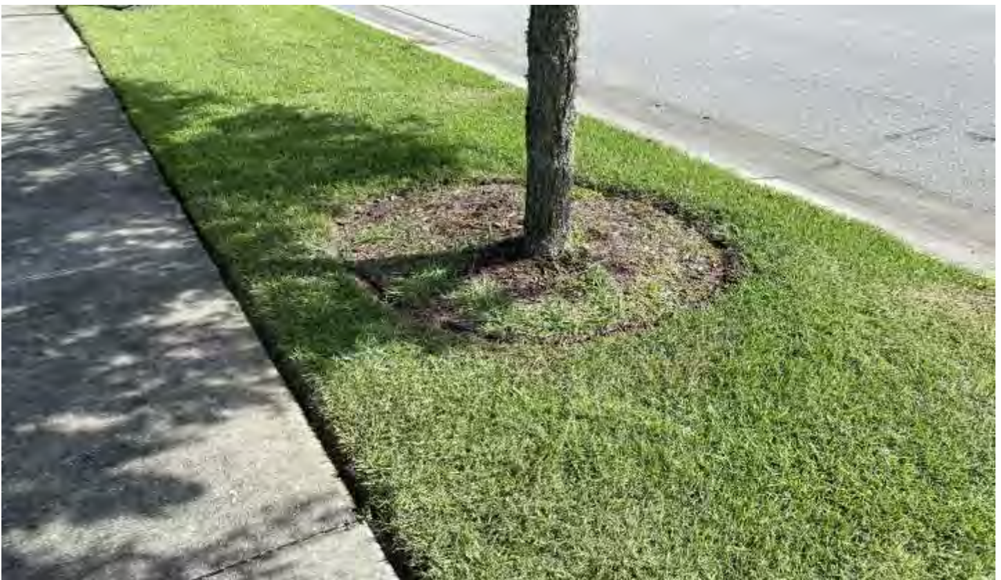
Tree wells need better detailing.
