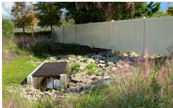
Figure 5: Riprap Placement at syphon inlet – North of fence
