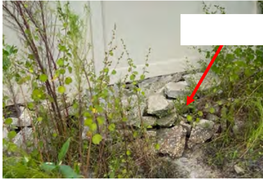
Figure 6: Riprap Placement south of fence
