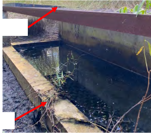
Figure 9: Syphon outlet – Close Up
