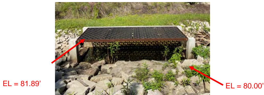
Figure 4: Syphon Inlet Configuration
